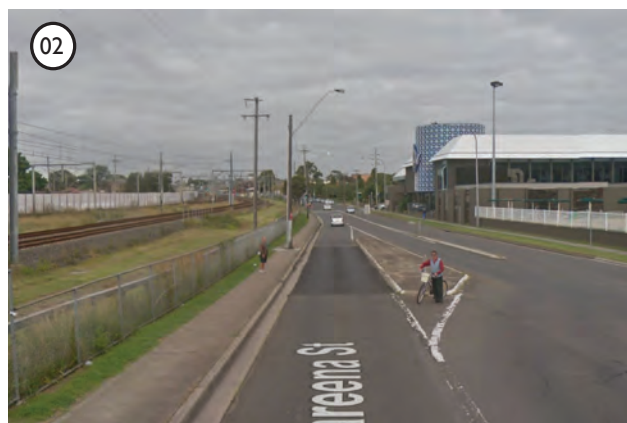
Eastern Boundary - Railway Parade, view due south
