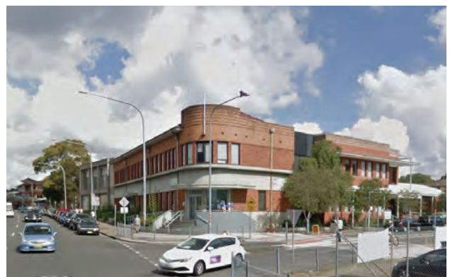
Local heritage item - Library and Civic Hall, Cabramatta (Source: Google Street view)
