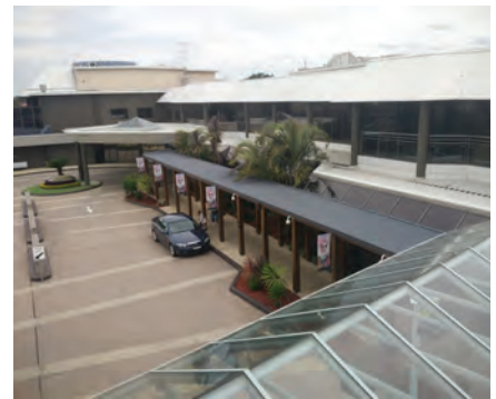
Existing club building in the southeastern part of the site.
