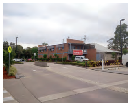
Existing brick building at the southwestern corner of the site.
